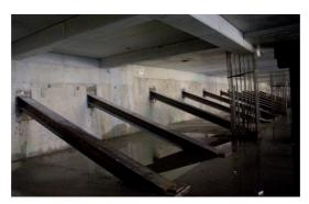
Fig. 1. View of the concrete slurry wall with supports and some construction elements that may obstruct surveying
